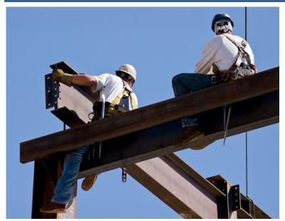
Hazard: Each year, falls consistently account for the greatest number of fatalities in the construction industry. A number of factors are often involved in falls, including unstable working surfaces, misuse or failure to use fall protection equipment and human error. Studies have shown that using guardrails, fall arrest systems, safety nets, covers and restraint systems can prevent many deaths and injuries from falls.
